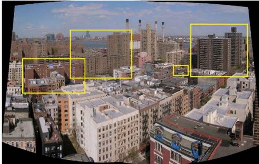
The Two Bridges/Beyond the Grid Community Microgrid Project Area, with participating sites outlined. (Microgrid Knowledge)
